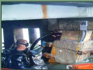
Equipment Operator 1 st Class (SCW/DV) Leroy Schnathorst pumps concrete in to formwork during pile restoration work.
