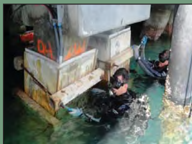
Construction Mechanic 3 rd Class Daniel Nichols and Builder 2 nd Class Keith Reed, prepare formwork for concrete placement.
