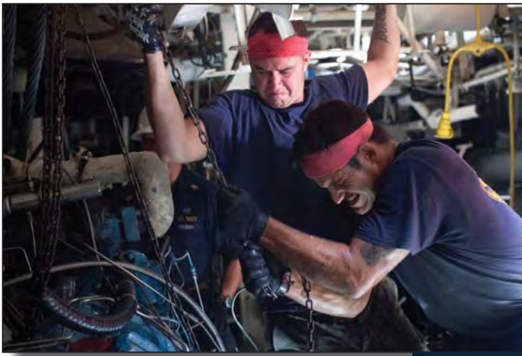
MDSU ONE divers rigging main engine for removal from Ex-USS Guardian.
