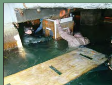
Equipment Operator 1 st Class James McVicar and Hospital Corpsman 1 st Class Ryan Irvine prepare formwork for concrete placement.
