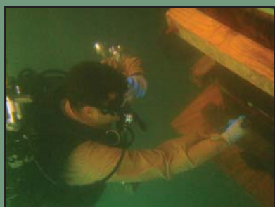
Hospital Corpsman 1 st Class (SCW/DV) Ryan Irvine uses a vibratory hammer during a pile restoration project to vibrate concrete within formwork surrounding a pile.
