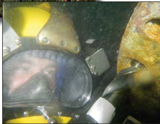
A member of the integrated JRMC/SWRMC Dive Team conducts underwater drilling onboard USS DENVER.
