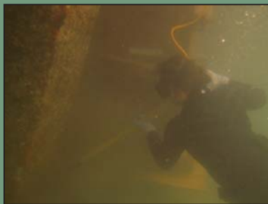
Steel Worker 2 nd Class (SCW/DV) Holly Ramirez prepares a pile at Joint Base Pearl Harbor's Hotel Pier for concrete form work by scrapping marine growth off with a heavy duty scraper.
